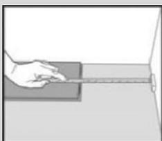
At the end of the first row, put a spacer  $\approx$ 15mm, to the wall and measure the length of the last plank to fit.
